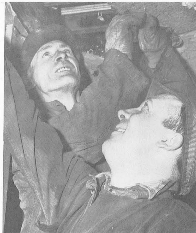
IT'S FATE--Sooner or later everything has to happen at Wayne. In this instance, two workmen are shown busily repairing a ceiling at Student Center. A pipe broke, flooding several rooms and sending surprised students scurrying for "high" land.
